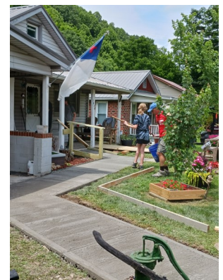
Completed Concrete Path
